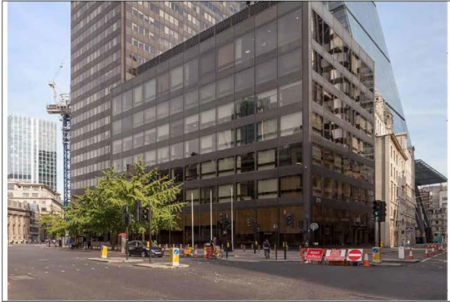
2. View north east from the junction of Gracechurch Street and Cornhill
